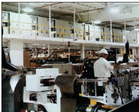
Control systems integration of entire production lines
